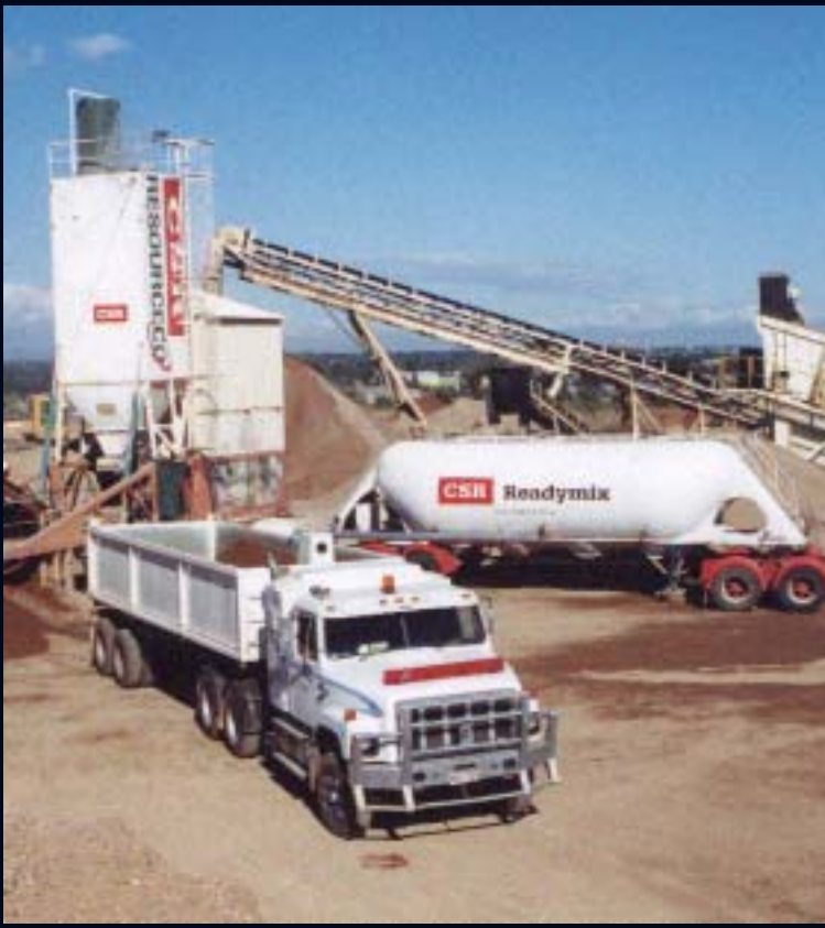
CSR Resourceco Cement Treated Aggregates Plant
