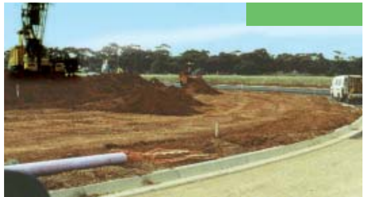
Recycled aggregates in use at Edinburgh Park
